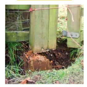
Posts rot at the ground line because conditions for decay are ideal at this point. Natures own natural waste disposal system for wood and leaves also happens to like eating your posts.
