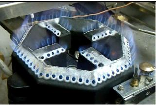
12. After burner installation, turn on the isolation gas valve and check for gas leak. Light up the burner and check if it has blue flame. For any abnormality found, follow the troubleshooting guide.
