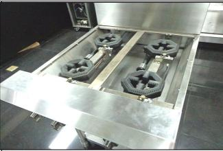
. Remove the trivets and knobs, and front control panel cover.
