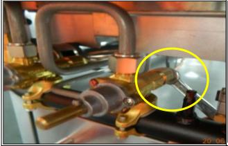
3. Disconnect the thermocouple from the safety gas valve.
