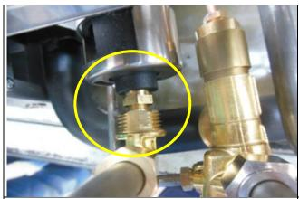
When installing the burner to the injector, make sure that the injector is fully inserted in the burner hole and that the injector is properly aligned.
