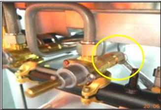
7. Reconnect the new thermocouple to the safety gas valve. Use 9mm spanner. Tighten the thermocouple up to 2.5N-m of torque. Tightening too much can cause the thermocouple to break and fail.
