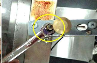
8. Reconnect the new thermocouple to the FDS. Then, open the gas isolation valve.
