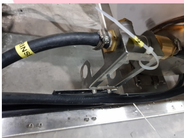
Image - 4: BOILER INPUT connection of the electric boiler
