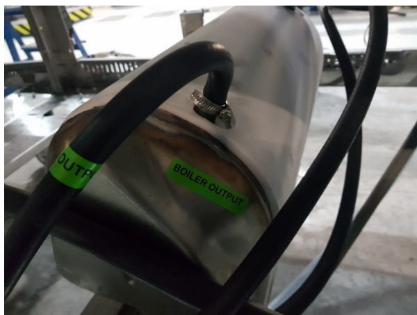
Image - 3: BOILER OUTPUT connection of the electric boiler
