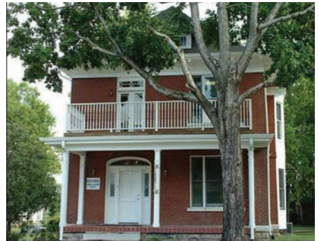
This is an older image of the Boyd House. It is in current need of major repair and has sustained significant damage to the exterior.
