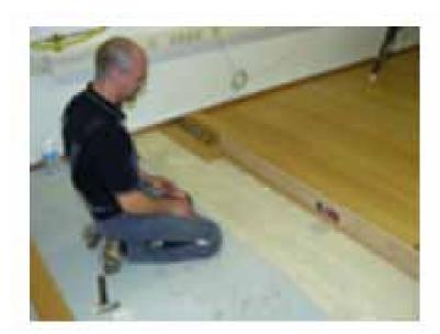
The installation is simple and the **fidbox**® is invisible to the naked eye. It takes separate readings of the temperature and relative humidity on the material surface and at the screed level.
