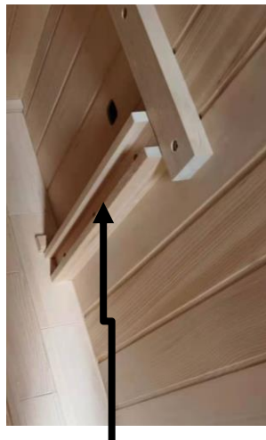
BENCH HEAT EMITTER PANEL Guides On Side Walls
