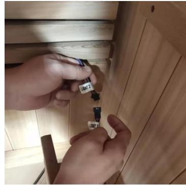
Rear Right – Corner Light Connection
