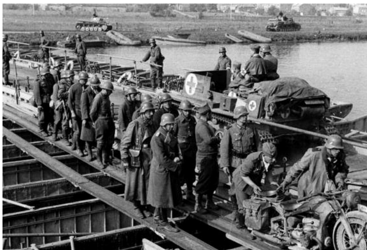
14 May 1940—1st Panzer Regiment crosses pontoon bridge with French prisoners over the Meuse at Floing, France. Bundesarchiv, Bild 146-1978-062-24 / CC-BY-SA 3.0
