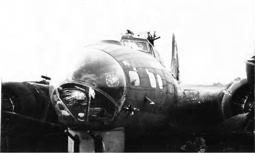
The nose and plexi-glass took numerous flak and 20mm hits by German fighters.
