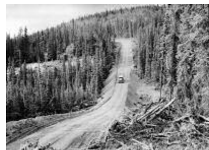
Alaska (Alcan) Highway between Edmonton, Canada and Fairbanks, Alaska
