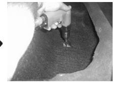
STEP 6: With a 1/2" drill bit. Drill a hole into the floor using the imprint in the wax square as guide.
