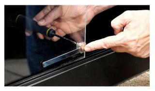
2. Before applying the security bars, first position the lock on the inner edge of the rear door panel. It's recommended to position the lock approximately one inch from the bottom. Once positioned, gently screw it into place. Use a screwdriver only, so that the screw is firm, but not too tight.
