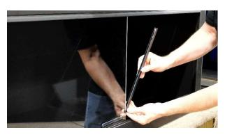
4. Once the sealant is applied, position the security bar on the inner edge of the rear door panel, starting from the bottom. Gently press the bar into place, leaving a small gap at the top for pane removal.
