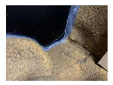
8. To finish, after the silicon has set, you can now go over the visible joins with a small amount of silicon and use the touch up kit to dab in the colored oxides to hide the joins and any silicon seams as well.
