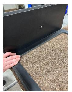
7. Begin by aligning Panels #1 and 2 as shown. We have already pre-drilled all the alignment holes for you in our workshop, so these parts will go together easily. It's important to make sure the ends are upright and flush with the bottom template. The drill holes in both panels will align accordingly.
