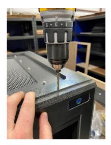
2. Through one of the front corners of Panel #1, drill straight into the top of the enclosure, using a 3/16" drill bit. It is important that you drill straight down, and that you only drill into your enclosure approximately 1/4". This is an important step to prevent the holes from drilling too deep and into the enclosure.
