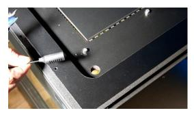
5. This is also a good time to drill the hole for the temperature and hydrometer probe. We recommend doing so on the cool side of your enclosure, using the space around your screen top. Once you have established where you would like the probe positioned, use a 3/8" drill bit to drill the hole, which will be just inside the template as shown.
