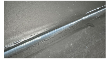
The finished seal!
