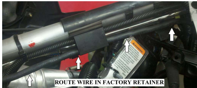
ROUTE WIRE IN FACTORY RETAINER
