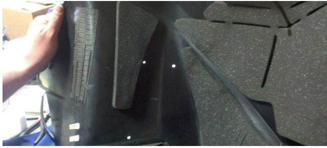
8. Cut the foam and remove on section.
