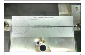
3. Drill a small pilot hole first then using an 1-5/8" hole saw, drill out the larger hole. Clean all shavings and rivet mandrels before continuing.
