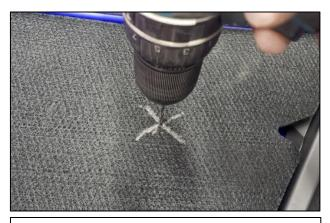
5. Using an 1/8" Drill Bit, drill a hole using the previous marks as shown. This hole is to be used as a reference hole only!
