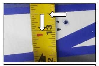
6. On the outside of your panel, measure %" forward and down from the previously drilled hole. Use a 1/8" Drill Bit to drill out this new pilot hole.
