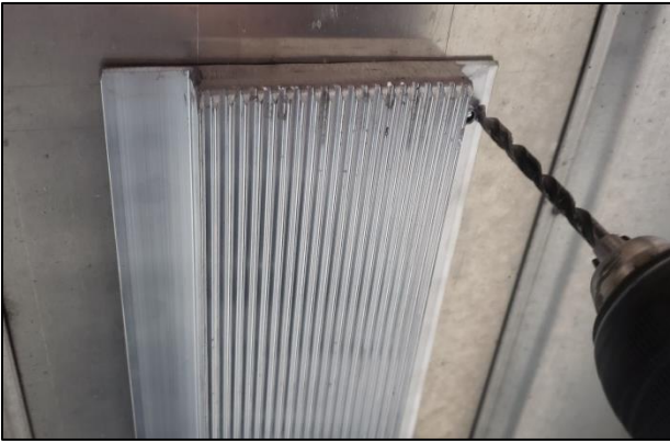
5. Be sure the Tunnel Cooler is centered in the tunnel. Drill a 3/16" hole on the side of the cooler, near the back of the Tunnel Cooler.
