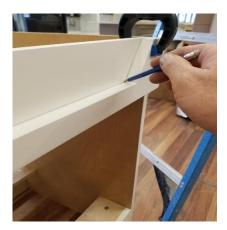
13) Remove the spring clamps and set the toe kick panel aside, then drill 5 - 3/16'' holes through the flat toe-kick panel inside the pencil line previously drawn. Re-clamp the decorative toe kick and attach with  $5 - \#6 \times 1/14''$  wood screws.
