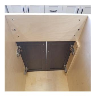
Rest a paint stick across the top of the cabinet doors for spacing and clamp the top face plate to the cabinet body. Use a pocket level to ensure that the face plate is level from side to side and check to make sure that the gap left at the top is the same all the way across the length of the face plate. Once the face plate is square and level, affix it to the cabinet with 4 - #6 x 1 1/4" screws from the back through the holes previously drilled, and repeat for the other side.
