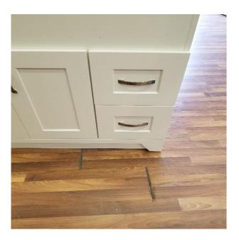
**IMPORTANT NOTE:** Your drawer faces will be loose to allow for adjustment at this point. After the cabinet is installed and leveled, you will need to square and level the doors and drawer faces again, this time making sure you permanently secure the face plates by driving 2 - #6 x 1 ½" wood screws through the 2 upper-most holes in the inside front face of the drawer box and into the back of the face plate, thereby ensuring the face plate stays square and cannot shift.
