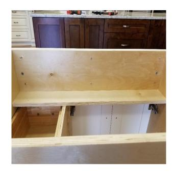
Remove the spring clamps and paint stick and your new 36" vanity is now complete and ready for installation. It is a good idea at this point to thoroughly vacuum out the entire cabinet to ensure that no sawdust or splinters from drilling can get into the drawer slides as over time they may potentially inhibit the proper operation of the slides and / or door hinges.
