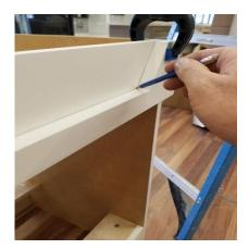
12) Remove the spring clamps and set the toe kick panel aside, then drill 5 - 3/16" holes through the flat toe-kick panel inside the pencil line previously drawn. Re-clamp the decorative toe kick and attach with  $5 - \#6 \times 1/14$ " wood screws.
