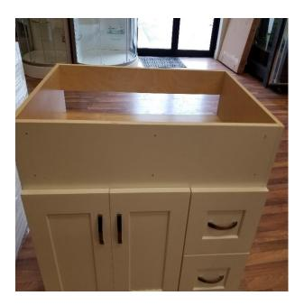
Rest a paint stick across the top of the cabinet doors for spacing and clamp the top face plate to the cabinet body. Use a pocket level to ensure that the face plate is level from side to side and check to make sure that the gap left at the top is the same all the way across the length of the face plate. Once the face plate is square and level, affix it to the cabinet with  $4 - \#6 \times 1 \%$  screws from the back through the holes previously drilled.
