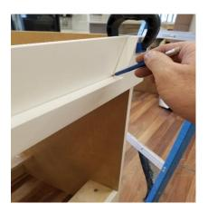
12) Remove the spring clamps and set the toe kick panel aside, then drill 5 - 3/16" holes through the flat toe-kick panel inside the pencil line previously drawn. Re-clamp the decorative toe kick and attach with 5 - #6 x 1/14" wood screws.
