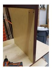
8) Locate the 2 side panels of the vanity, they should be the largest remaining pieces with finished outsides, place them finish down and spine to spine on your work surface and affix steel locking pins into all available white receptacles in both side panels. Then locate the pilot holes in the side panesl and affix the remaining 6 drawer slides to the panels using #6 x 5/8 wood screws.
