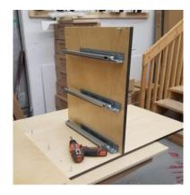
5) Locate and dowel the 2 short front braces that will attach the side panels to the drawer gables and affix them to the drawer gables using one steel locking cap per brace. Ensure that the finished edge of each short brace faces forward.
