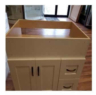
Rest a paint stick across the top of the cabinet doors for spacing and clamp the top face plate to the cabinet body. Use a pocket level to ensure that the face plate is level from side to side and check to make sure that the gap left at the top is the same all the way across the length of the face plate. Once the face plate is square and level, affix it to the cabinet with  $6 - \#6 \times 1 \%$  screws from the back through the holes previously drilled.
