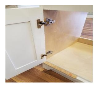
14) Use the various adjustment screws on the body of the hinges (6 way adjustment) to make sure that the doors are evenly spaced, square and level, and attach each handle to the door using the screws provided in the package with the handle.
