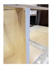
6) Locate the 2 side panels of the vanity, they should be the largest remaining pieces with finished outsides, place them finish down and spine to spine on your work surface and affix steel locking pins into all available white receptacles in both side panels. Then locate the pilot holes in the right-most side panel and affix the 2 drawer slides to the panel using #6 x 5/8 wood screws.
