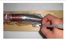
2. Wire the light based on the wiring diagram. Feed wires back into the hole and use silicone sealent around the wires to prevent any ingress of water. For added protection use silicone around the end caps.
