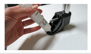
**4.** Using #10 screws (not provided), install the end caps in the pre-drilled holes. Note: The innermost holes toward the door must be used at all times, it is recommended that all four holes be used on each end cap. If there is no backer than you may need to use a bolt, large washer, nut and plate (not provided).
