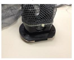
3. Use the shower cup screw holes as a pilot and pre drill holes with the 7/64" drill bit. Drill the top hole first and install the screw. Now align the cup and drill the bottom holes. Do not over tighten these screws. Screw this in by hand or turn the electric screw driver to low torque setting.
