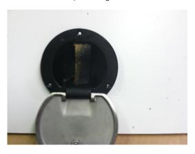
Ensure either ITC screws provided are used or #6 screws. Larger screws could cause damage to the plastic cup.
