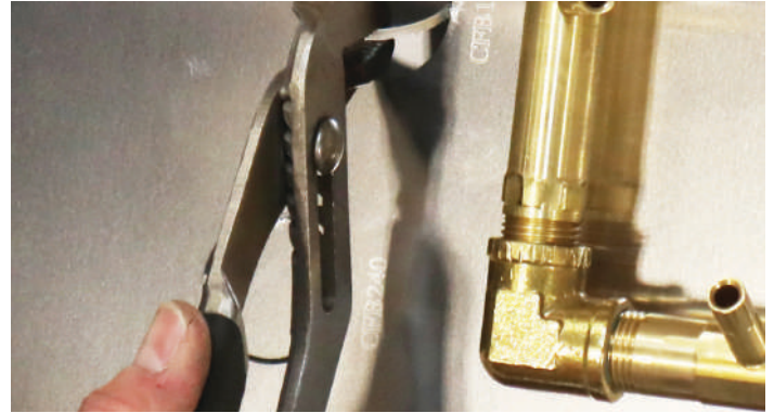
Photo 2: Breaking the Knockouts
