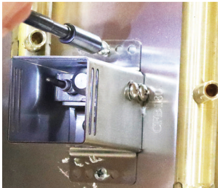
Photo 5: Securing the Pilot to the Plate/Pan
