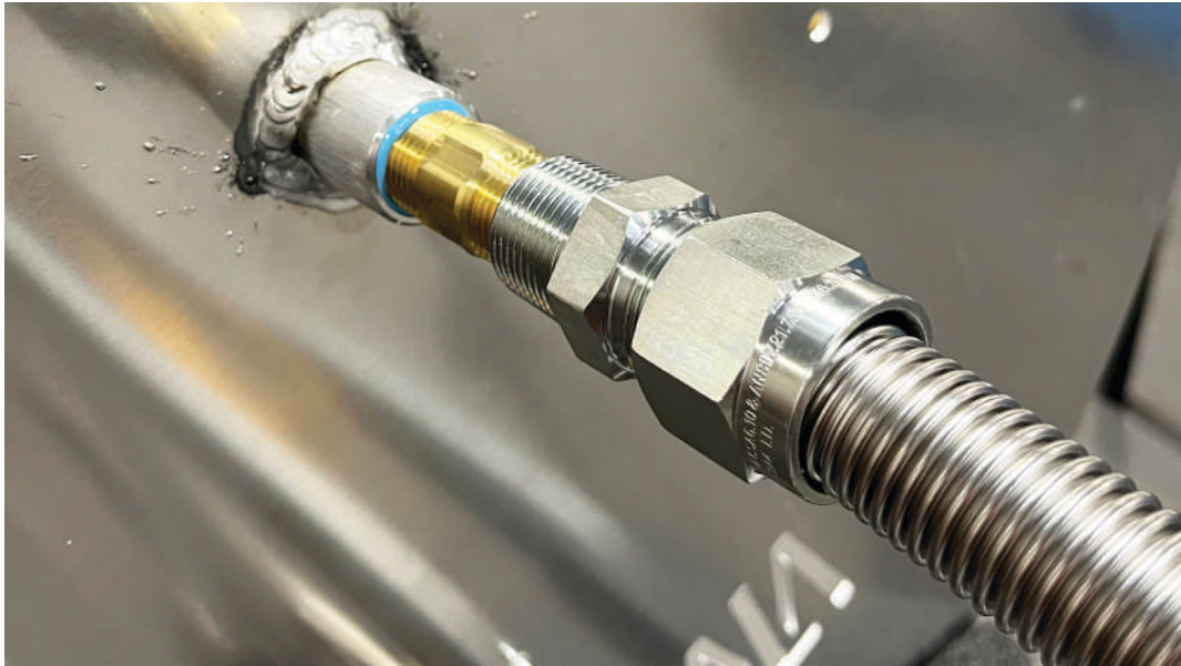
Photo 18: Connecting the Flex Line
