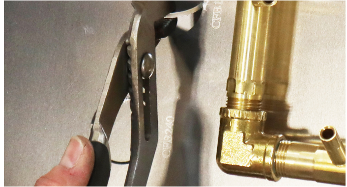
Photo 2: Breaking the Knockouts
