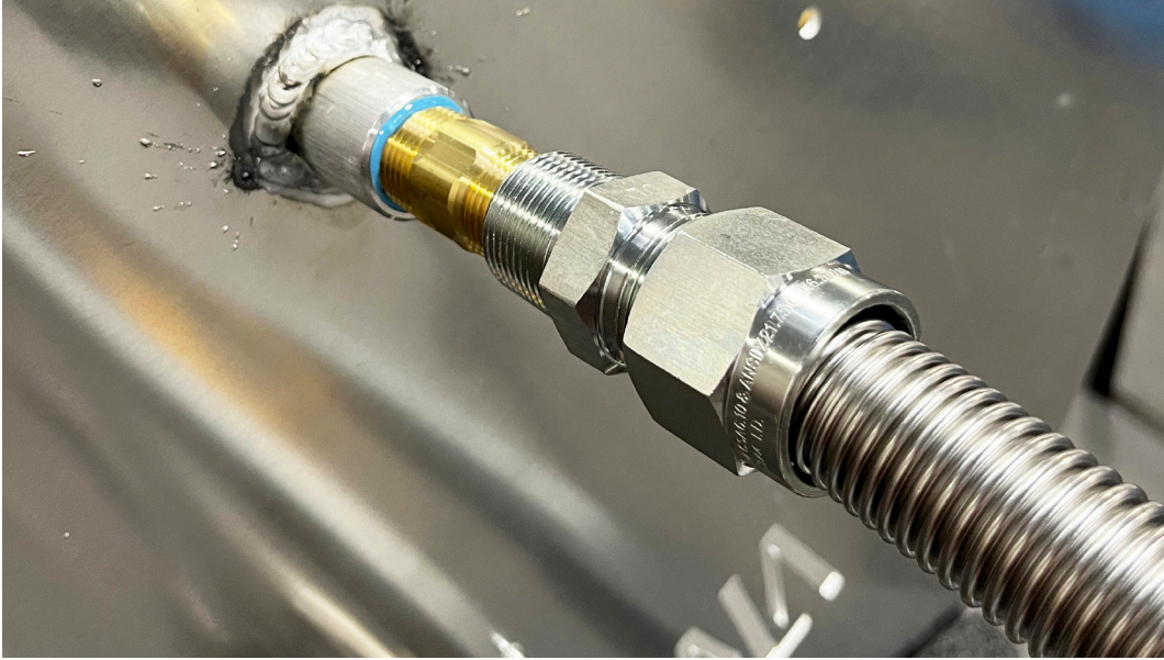
Photo 18: Connecting the Flex Line
