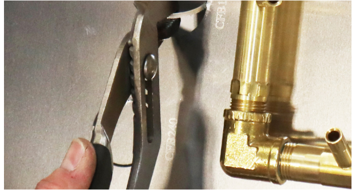
Photo 2: Breaking the Knockouts
