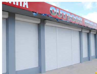
Commercial Store Fronts
