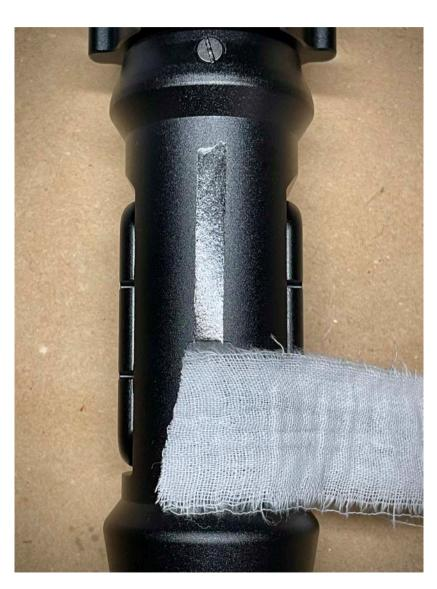
Now to apply the first part of the wrap. Provided in the wrap kit are three different white fabrics, this one stands out as it is more of an open weave material.
