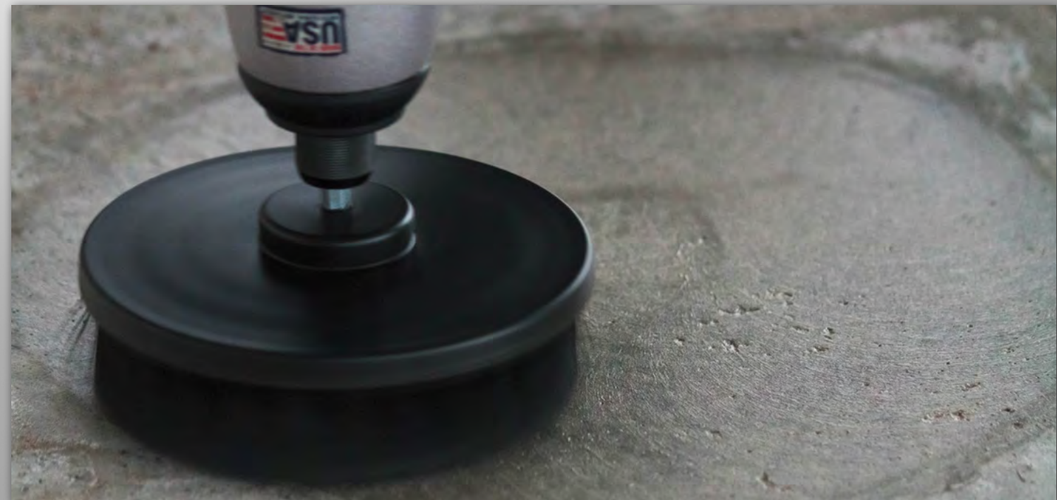
Ultra Stiff 5 inch brush cleaning concrete.
