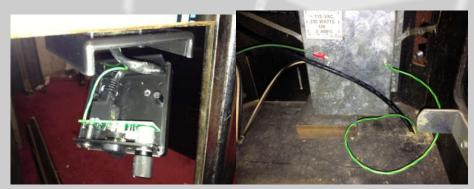
Secure wire to ground stud on power box. Continue with Back box board installation.
