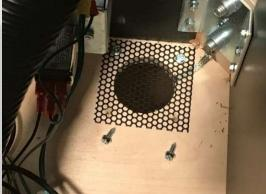
Fish the 3.5mm subwoofer cable through the vent hole in the bottom of the cabinet.
