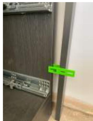
As you can see in this image, the U-Scribe Jig are holding the filler panel over the front of our cabinet, our cabinet on this project is 18mm, so now we are offset by 18mm, the reason we call this the “Off Set Method”
