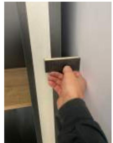
Now using the block positioned against your wall, Simply scribe a line onto your filler panel, the block is following the contour of your wall adding the perfect image onto your filler material, U-Scribe Jig acting as your #3rdhand
