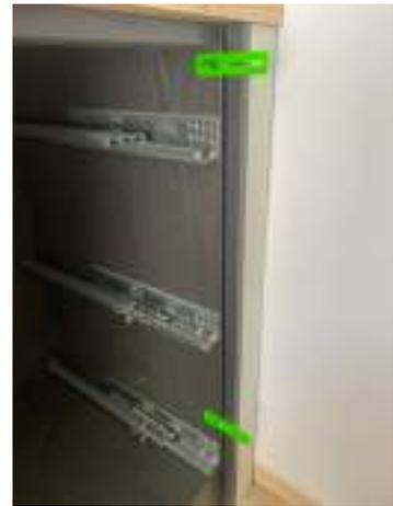
Using an off cut block of the same thickness of your cabinet or material (18mm in this case) position it against your wall and mark down your wall with a pencil or marking knife, you are drawing the perfect image directly onto your filler
