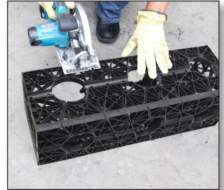
Cutting the module with a circular saw
