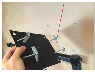
Step 8 - Slightly pull each corner of the bracket towards you and tighten each bolt until there is about 1/2" of space between the wall and the bracket. Move to the next bolt, until all bolts have the same spacing. Continue pulling the bracket and move around all bolts again until plate is flush to the wall.
