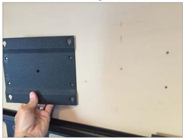
Step 6 - Insert toggle bolts and attach hinged wing nuts so the tip of the bolt passes the end of the nut.
