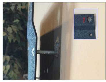
Step 9 - OPTIONAL - use 1 5/8" wood screw for remaining "non toggle bolt" holes.
