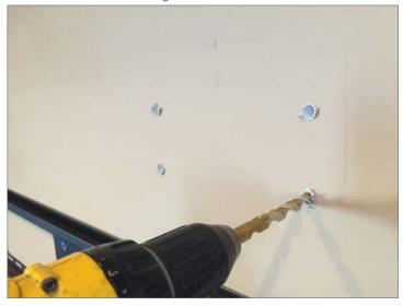
Step 7 - Make sure that wall mount bracket is mounted so that the notch of the DVD mounting hole is facing down (1). Insert toggle bolts into wall and push all the way in so wing nuts open.
