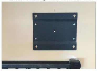
Step 5 - If you are fastening the bracket to drywall, use a 1/2" drill bit to drill through the wall where no studs exist.
