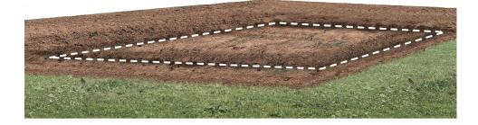
Step 2 Prepare the foundation according to the greenhouse size (length & width). As for the depth, it should be at least 4 inches under the ground surface.
