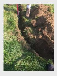
Place and Connect Airline in the Trench Place a single run of 1" Direct Burial or PVC Pipe (sold separately) in the trench from the cabinet location to the pond's edge.
