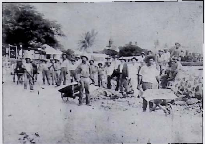
Turn of the century sea wall construction on Alii Drive. Back in the days when Kailua was only a cattle shipping town. Photo courtesy of the Kona Historical Society.
