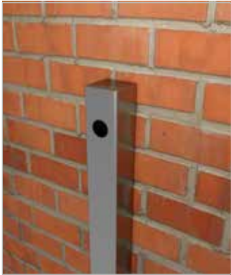
1 Drill a 25mm diameter hole through front wall of post
