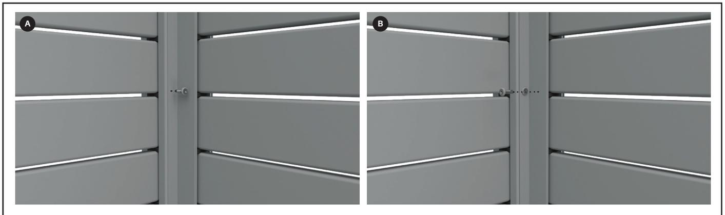
10 A) Move F channels out against rear side posts and drill 3 x 3mm pilot holes through F channel leg into rear post at the top, middle and bottom. Screw fix with 3 x 10Gx16mm wafer head screws. Repeat on other side. F channel is now screw fixed to rear posts at both sides.
