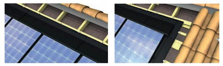
Place the precompressed seal on the flashings around the area on the lateral and upper parts.
