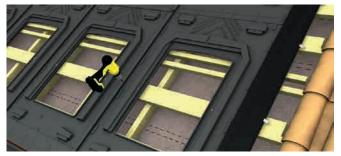
• For end clamps, pre-drill through the flashing, the frame's corrugation and the wedges.
