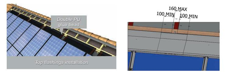
In the same way, place the corner flashings, having applied beforehand a PU glue joint on the overlapping zone of the top flashing. (Overlapping at least 100mm)
