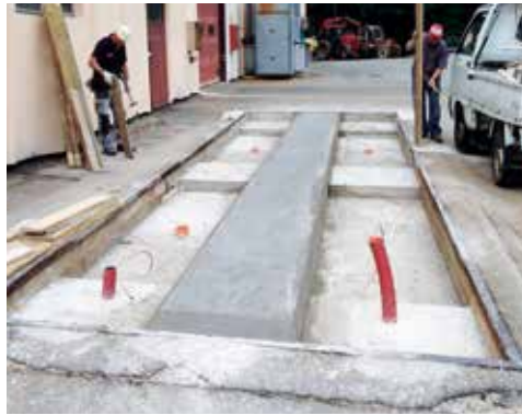
Example of a recycled existing pit
