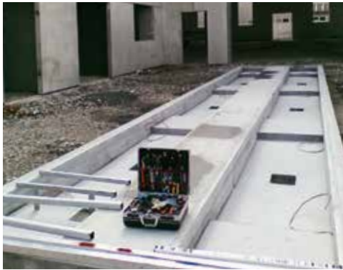
Example of a new installation
