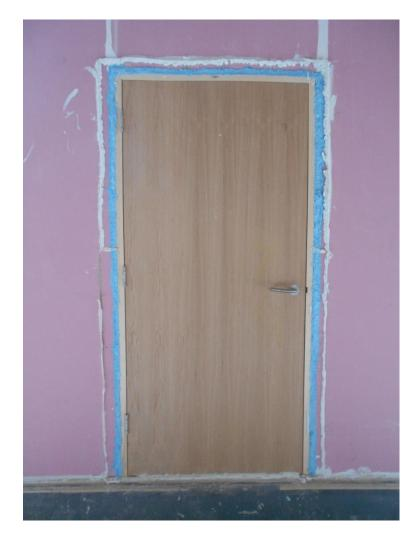
The doorset (which was not tested), consisted of a Vicaima GDC leaf, fitted in a softwood frame. The overall frame dimensions were 1000mm wide x 2100mm high x 100mm deep and the leaf dimensions were 926mm wide x 2040mm high x 44mm deep.
