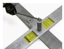
Step 11: Using the tightening bar, secure the eyebolt firmly in place.
