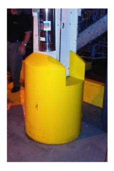
Bare Post before Column Sentry Concrete Wrap protection product is installed. You can see how vulnerable it is to forklift collision damage.
