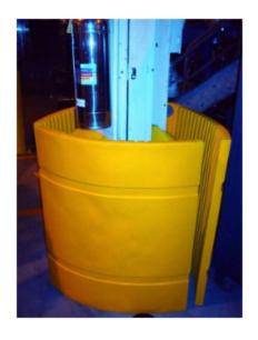
Position wrap protection panels around the concrete post.
