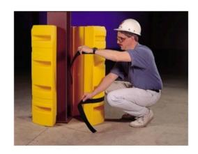
First, place the product around the column and extend the straps around the installed protector. Finally, press the hook and loop straps together for a tight fit.
