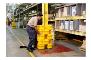
Slide those "halves" toward each other, sliding the parts together or apart, until it fits the column tightly.
