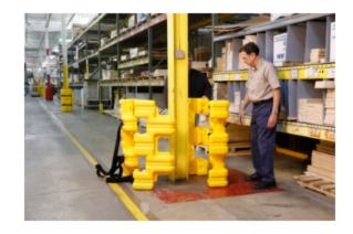
Position the 4 pieces of the Column Sentry FIT around the column. Slide 2 each together, until you have 2 equal sides.
