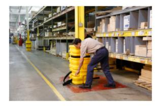
Wrap the finished column protector with the included 2-sided Velcro straps.
