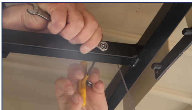
STEP 4F: Affix and tighten 10/32 Lock nuts using 1/8" allen wrench and 3/8" crescent wrench.
